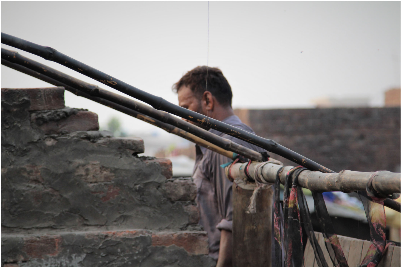
Figure 3. Strips of old cloth fastened to pieces of wood form the structure of a residential jhuggī (hut), Lahore, Pakistan, July 2015. (Waqas H. Butt) [This figure appears in color in the online issue]
